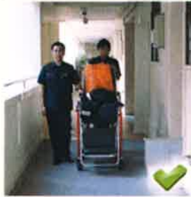
Ambulance crew and wheel chair bounded person requires at least 1.2m clear width for access. 救护人员和使用轮椅的人士需要至少1.2米的畅通空间才能顺利通过。
