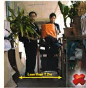
Obstruction to emergency crew access due to constricted corridor. 被阻碍的走廊阻碍救护人员的出入。
